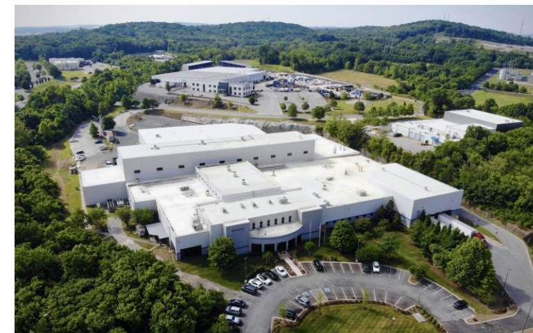
The expanded forming plant in Nashville, USA.
