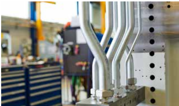
Pipework for the press with subsequent assembly of the infeed and outfeed
